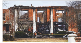
The day after: The remains of the building's Doric columns.
